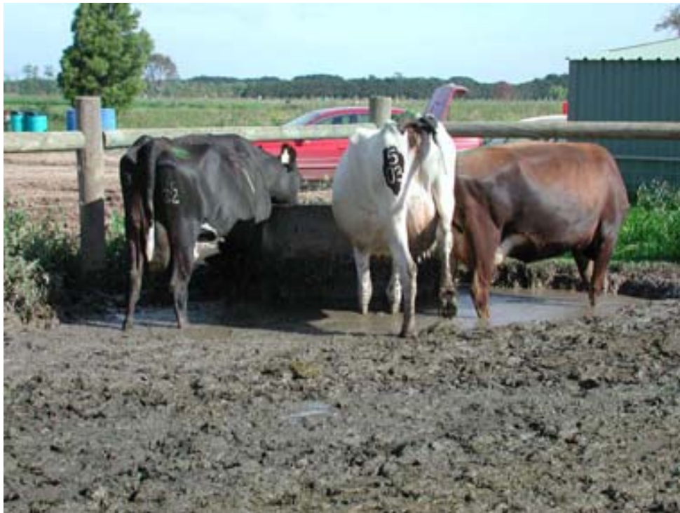
An area around a water trough which is in urgent need of repair. Such wet muddy areas will predispose to lameness.
